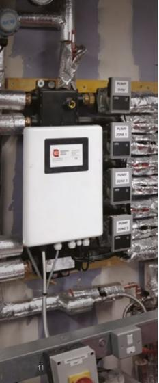
The fully pumped manifold combines a hydraulically separated low loss header with zone distribution, greatly reducing installation time and cost.
